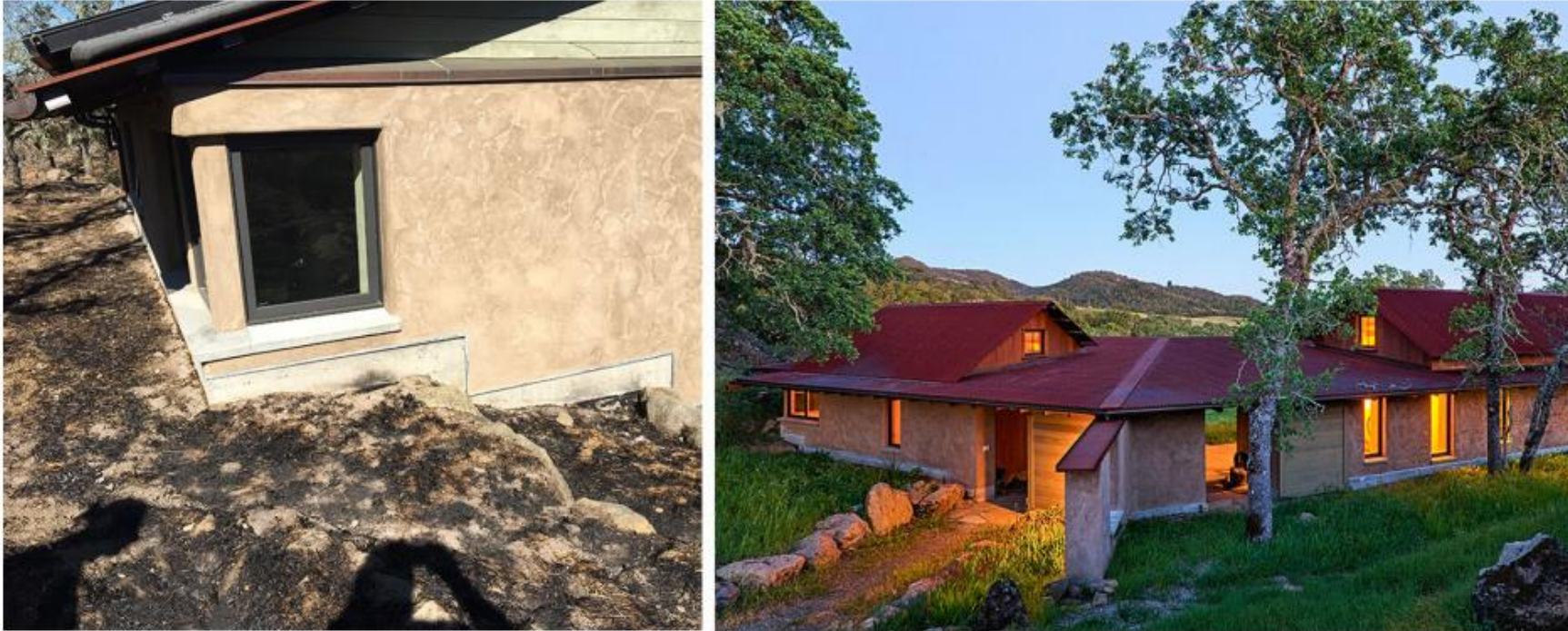
fig.1. Norrbom Road Strawbale Home - fires burned to the foundation on but not up the walls.
